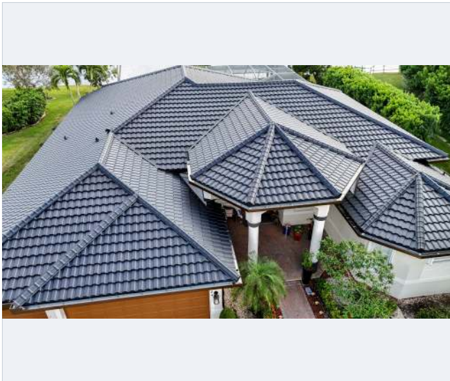
Worthouse DURA Raven Black — Florida installation
