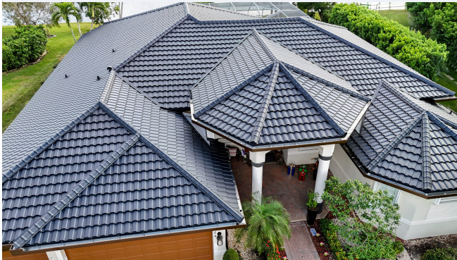
Worthouse DURA Raven Black — Florida installation
